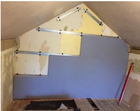
Once the isolation bars and clips are securely fixed the next step is to install the first layer of acoustic plasterboard. The first layer of acoustic plasterboard should be 19mm thick and shall align seams between sheets on the centerline of the horizontal channels. Ensure a gap is left around the linings to decouple the layer.
