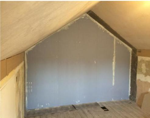
For the second layer of plasterboard ensure there is a gap left around the linings so the system is completely floating. The perimeter gap can be filled with our flexible acoustic sealant. All potential sound leaks such as gaps around outlets, window or door frames, pipe penetrations and the like are sealed with a flexible, non-hardening acoustic sealant.
